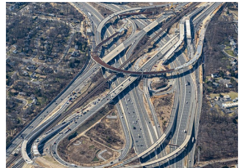
Structural Steel 2023 POY Class III Williams Steel Erection Co., Inc. Transform 66, Fairfax & Prince William Counties, Virginia
